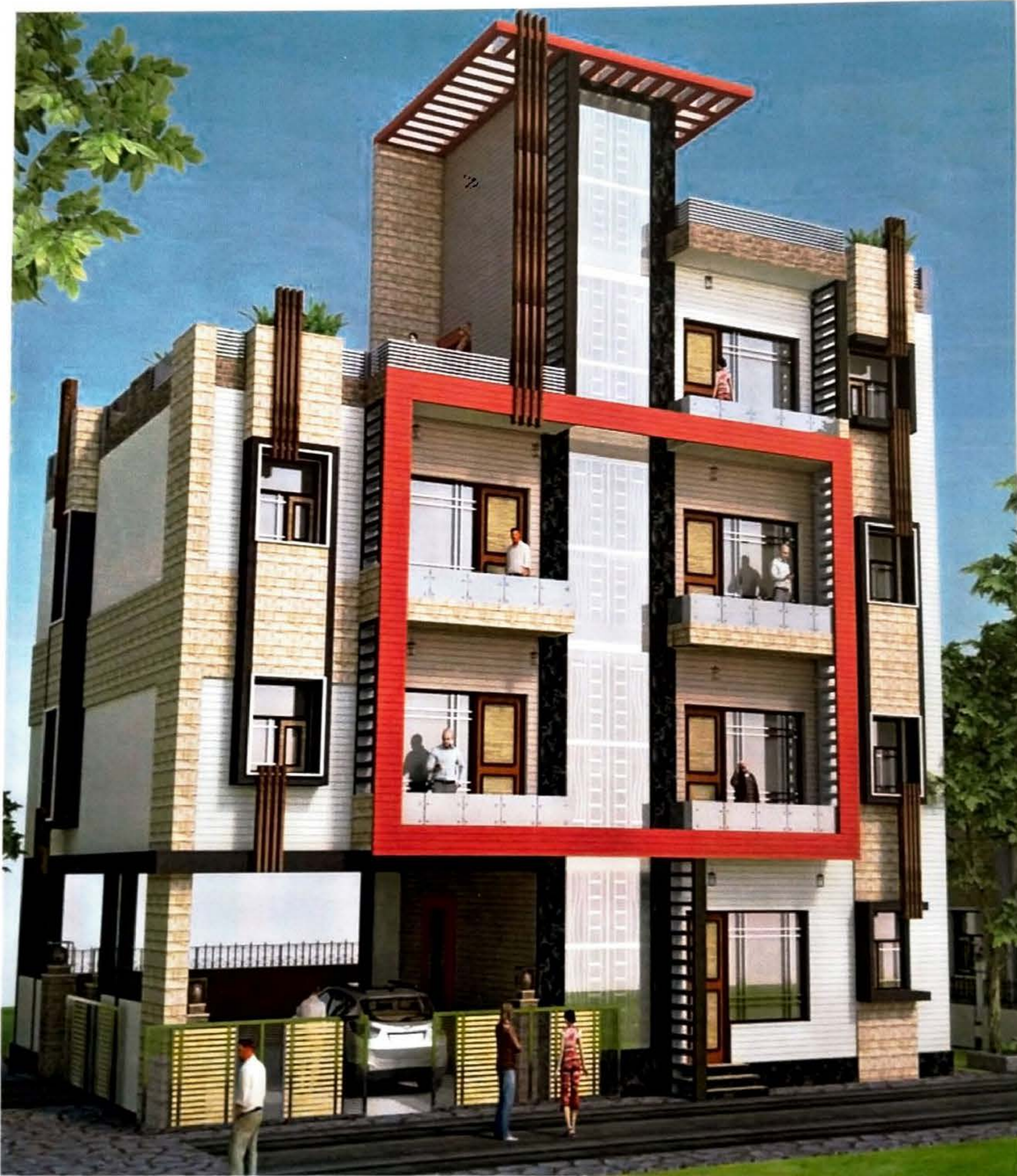
KRISHNA HOMES - 4 MULTISTORY BUILDING AT BLOCK NO. 54 THDC COLONY, DEHRAKHAS, DEHRADUN (AS A DEVELOPER)
