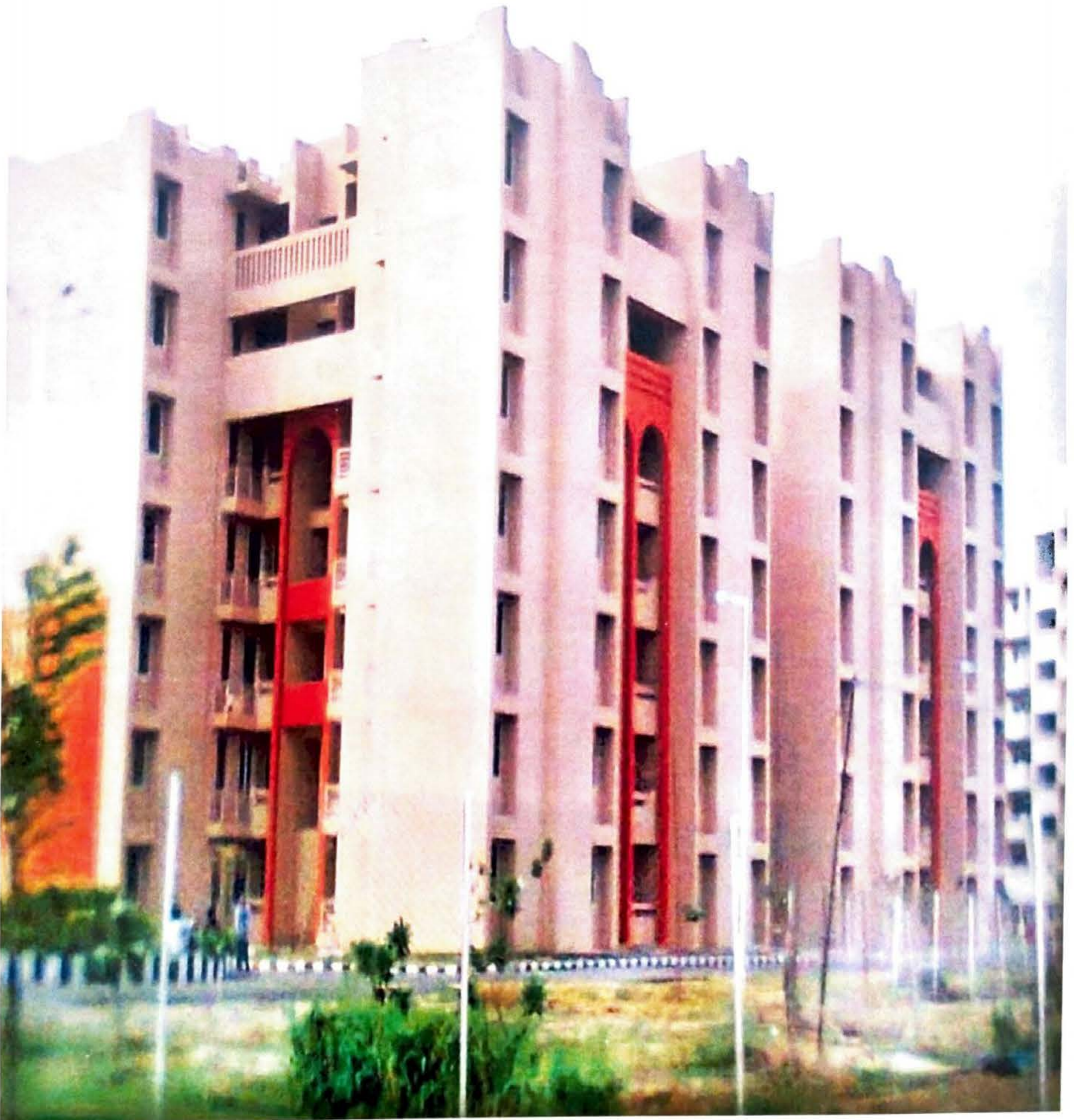
GROUP HOUSING PROJECT AT ROSHANABAD, SIDCUL, HARIDWAR (HERO GROUP)
