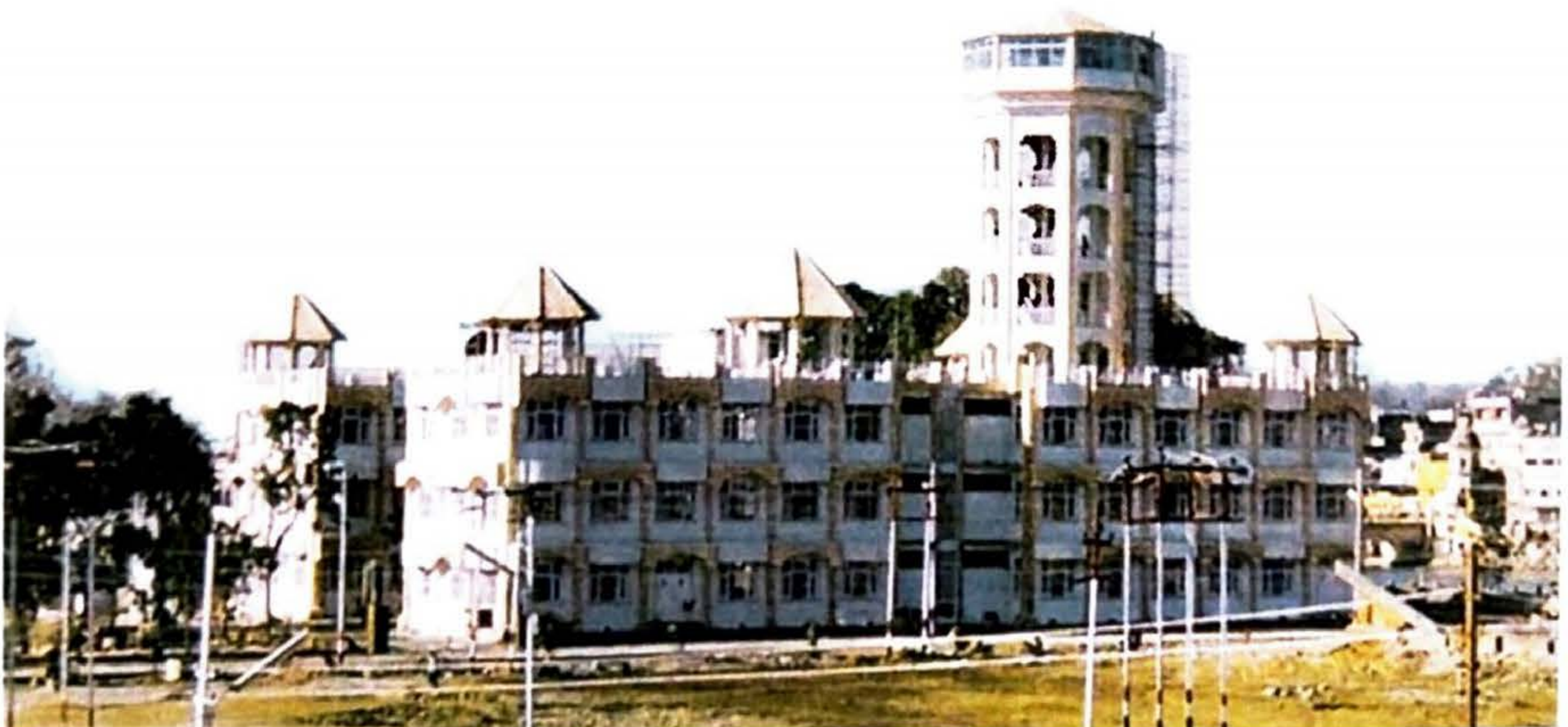
POLICE CENTRAL CONTROL ROOM AT LALJIWALA, HARIDWAR
